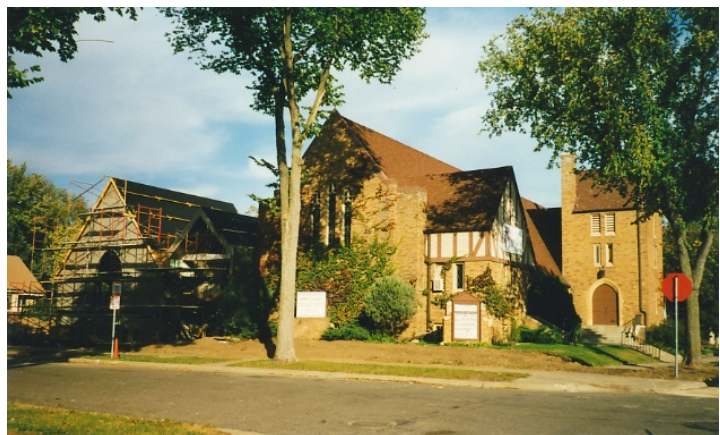
Construction of the 1998 building addition
