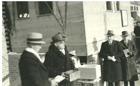
Laying the cornerstone on December 28, 1941.
