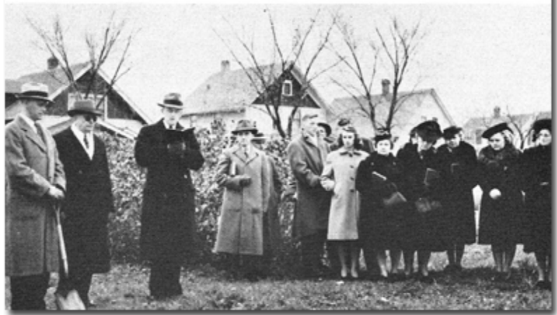
Breaking ground for the church building, November 9, 1941. Pastor Freedholm, Chairman Ezra Oberg, and Contractor Earnest Hultquist officiated.
